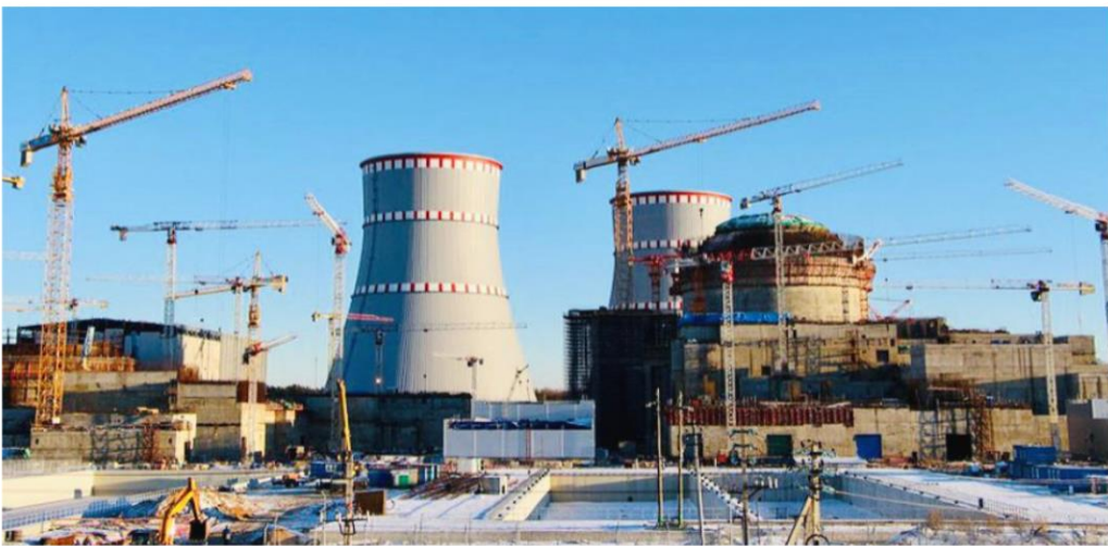
Rooppur Nuclear Power Plant
