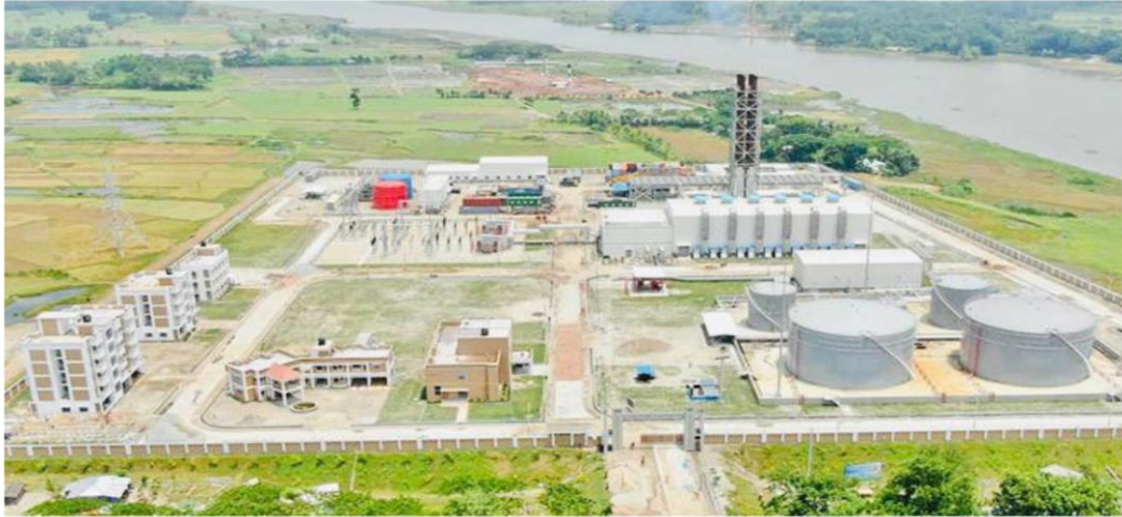
MadhuMoti Power Plant
